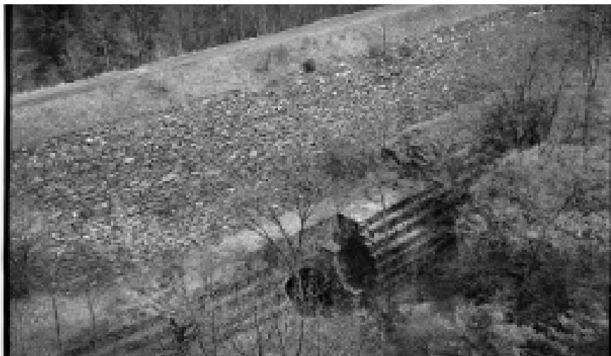
Mid-1960s Mill River Culvert
