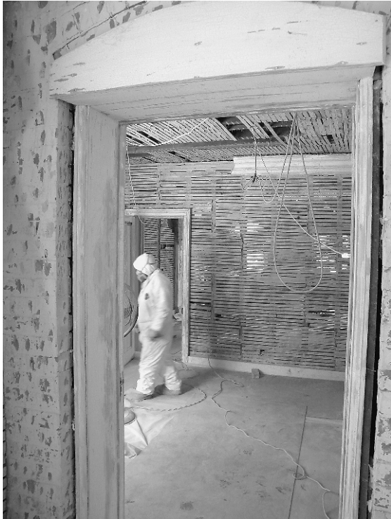
This painted doorway is upstairs and part of the later addition to the Keeper's House. The doorway was constructed using an exterior window frame, with its arched lintel mirroring the shape of the construction of the exterior windows of the original house. The workman is wearing a protective suit in case the paint he is removing contains lead.
