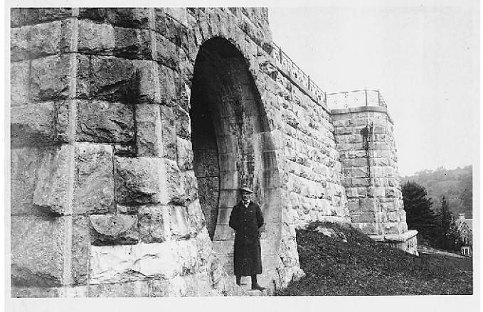
A 1902 photo of an intake portal at the site of the new gatehouse, similar in size and shape to the New Croton Aqueduct tunnel. The portal awaits the rising waters of the enlarged Croton Reservoir. Photo courtesy of the U.S. Geological Survey.
