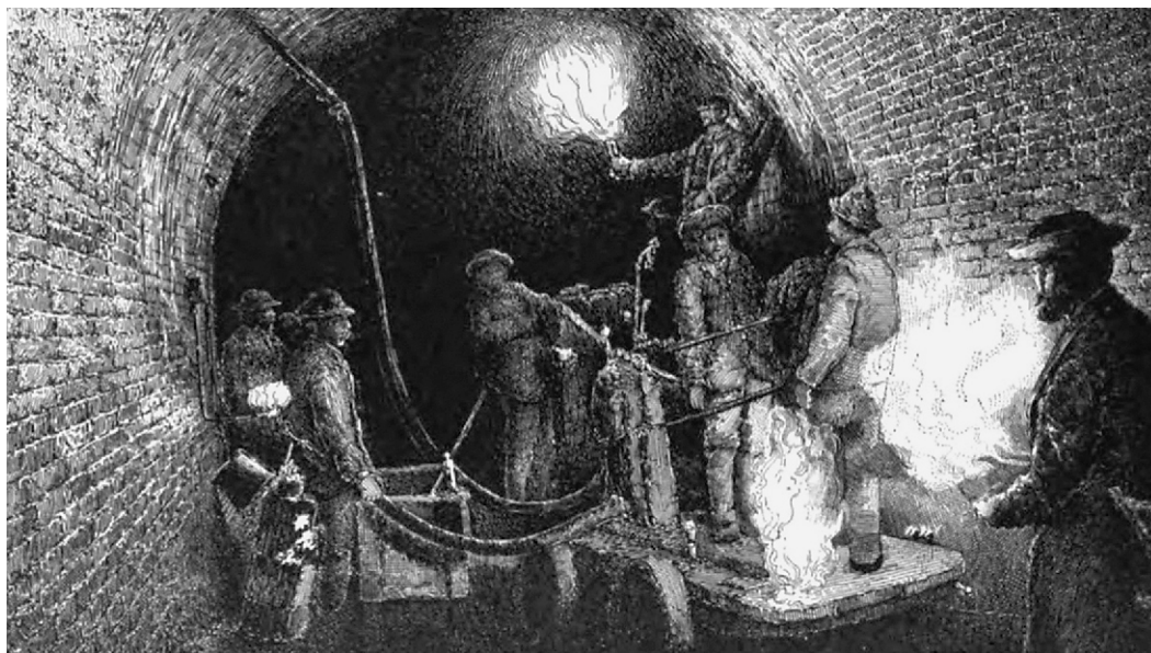
An illustration from an 1895 report to the Aqueduct Commissioners. Note the brick arch, torch and workers compared with the size of the tunnel.
