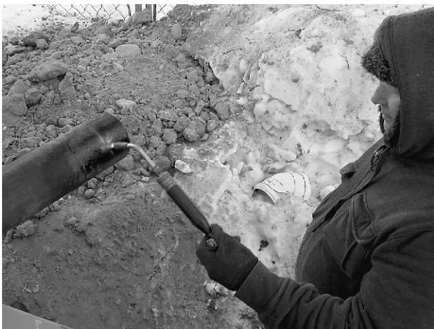
A plumber working outdoors at the Keeper's House in the extreme cold. Plumbers have been making final pipe connections from the waste line to the sewer.
