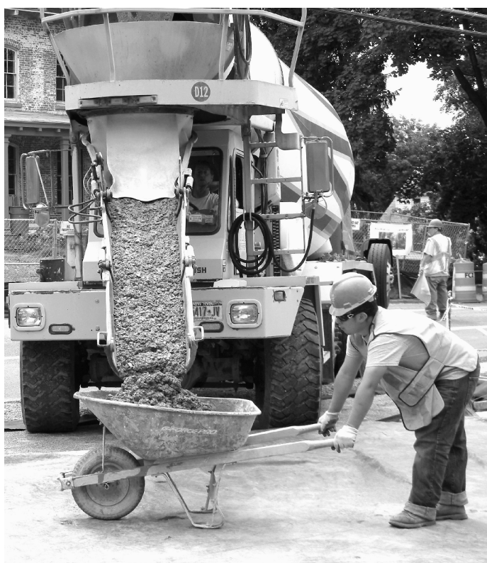
Concrete is delivered to a worker for pouring into the curb forms of the new parking lot for visitors with disabilities across the street from the Keeper's House.
