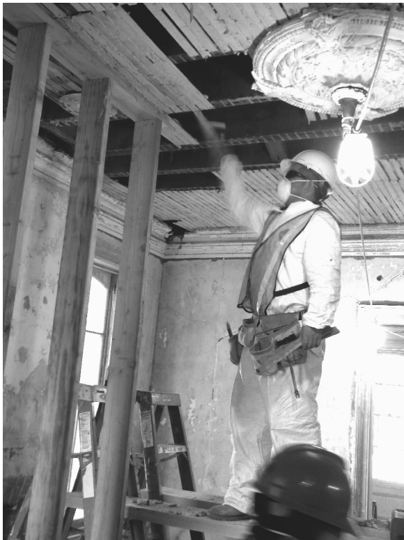
A worker removes old ceiling lathe in Room 2 in preparation for repair of a rotted beam.
