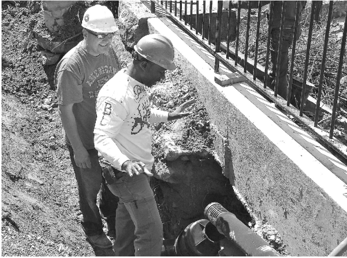
Site supervisor, Roger Moore, directing the installation of a new drainage pipe system for the top of the bridge.
