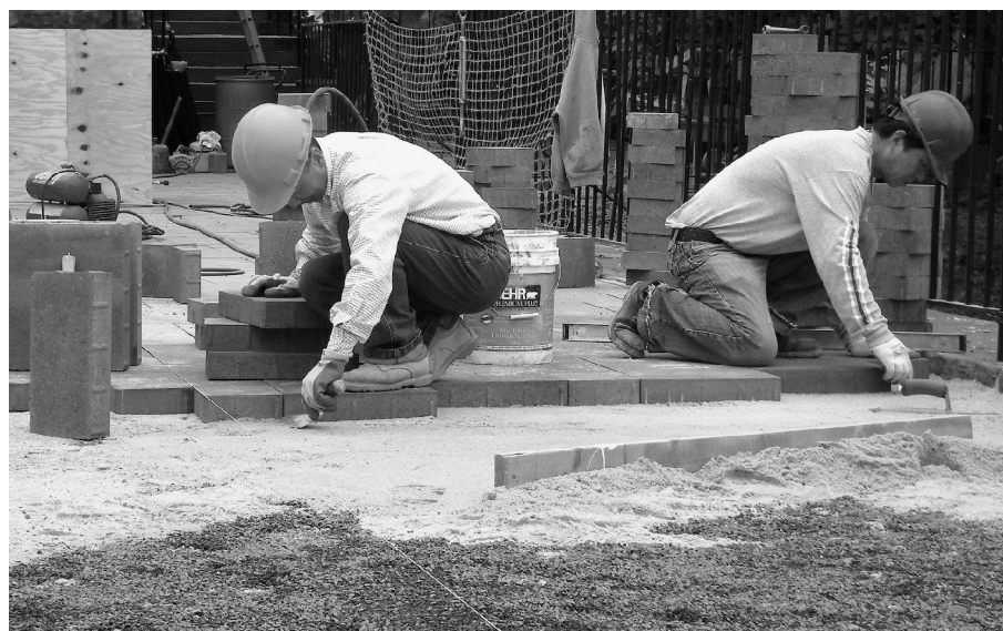
Two masons work on the walkway cement pavers.
