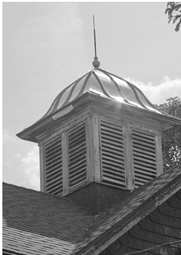
The gleaming new copper cladding on the cupola of the 1880s Aqueduct barn at Walnut St. in Dobbs Ferry. The barn is used by the State Parks trail maintenance crew. (Photo courtesy of Anne Marie Leone/Rivertowns Enterprise)
