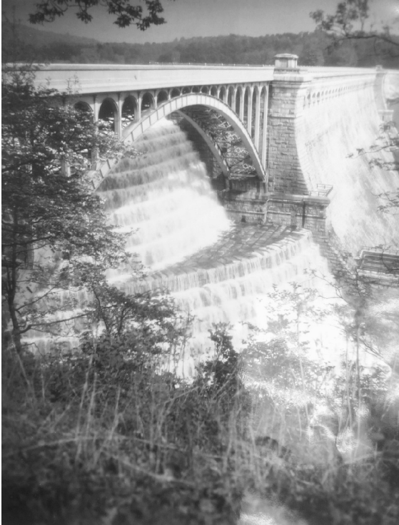
The entire structure of the New Croton Dam is of natural masonry. Almost all dams built afterward had large amounts of cast concrete block in addition to stonework. (Photo courtesy of the Croton Historical Society)
