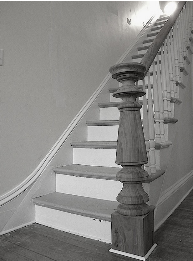
Rebuilt staircase and wall of entrance hallway. The formerly missing newel post was fabricated from reference photos taken at the Ossining KH, recently rediscovered as a mirror image of the house design in Dobbs Ferry. Numerous balusters were made to match the surviving ones on the bannister.
