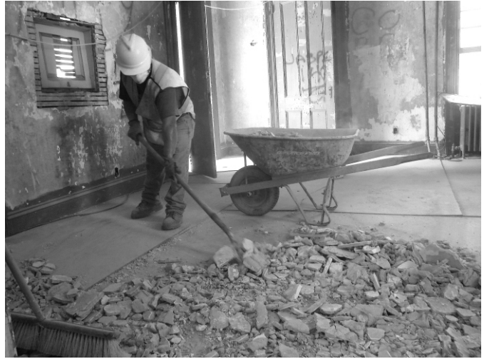
In 2014 a worker shovels plaster rubble from Room 2 downstairs. All the ceiling and wall plaster was removed from this room, then replaced with new sheetrock and plaster. A weak ceiling joist was reinforced and new electric lines and heating conduits were added while the ceiling was open.
