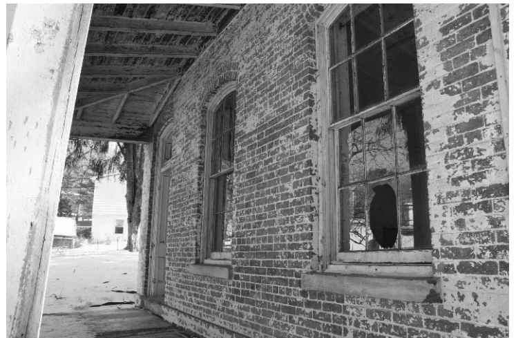
Top and bottom: A 2007 view of KH showing the dangerously sagging front porch structure, broken windows and peeling paint. The Friends were allowed to rebuild the porch structure as a separate project before the KH renovation. All photos on this page by E. Zazzera.
