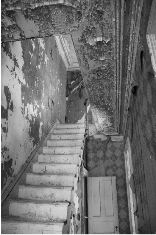
A 2007 view in the entrance hallway without staircase bannister, showing interior crumbling plaster, much of which had to be removed to bare brick and then rebuilt due to 40 years of roof leaks.
