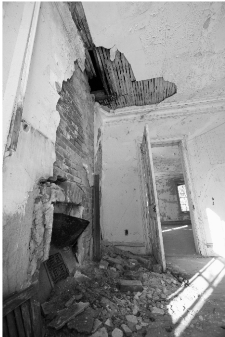
A 2007 view of foot-deep pile of fallen plaster and brick rubble on the second floor under a section of deteriorated exterior brick wall through which the sun shone and the rain and snow fell. The rubble remained in place long enough to rot the floor section beneath it.
