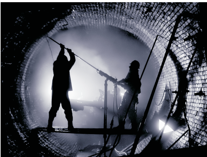
Rock drilling underway to connect the New Croton Aqueduct to the Croton filtration plant. (Photo courtesy of NYC Dept. of Environmental Protection)
