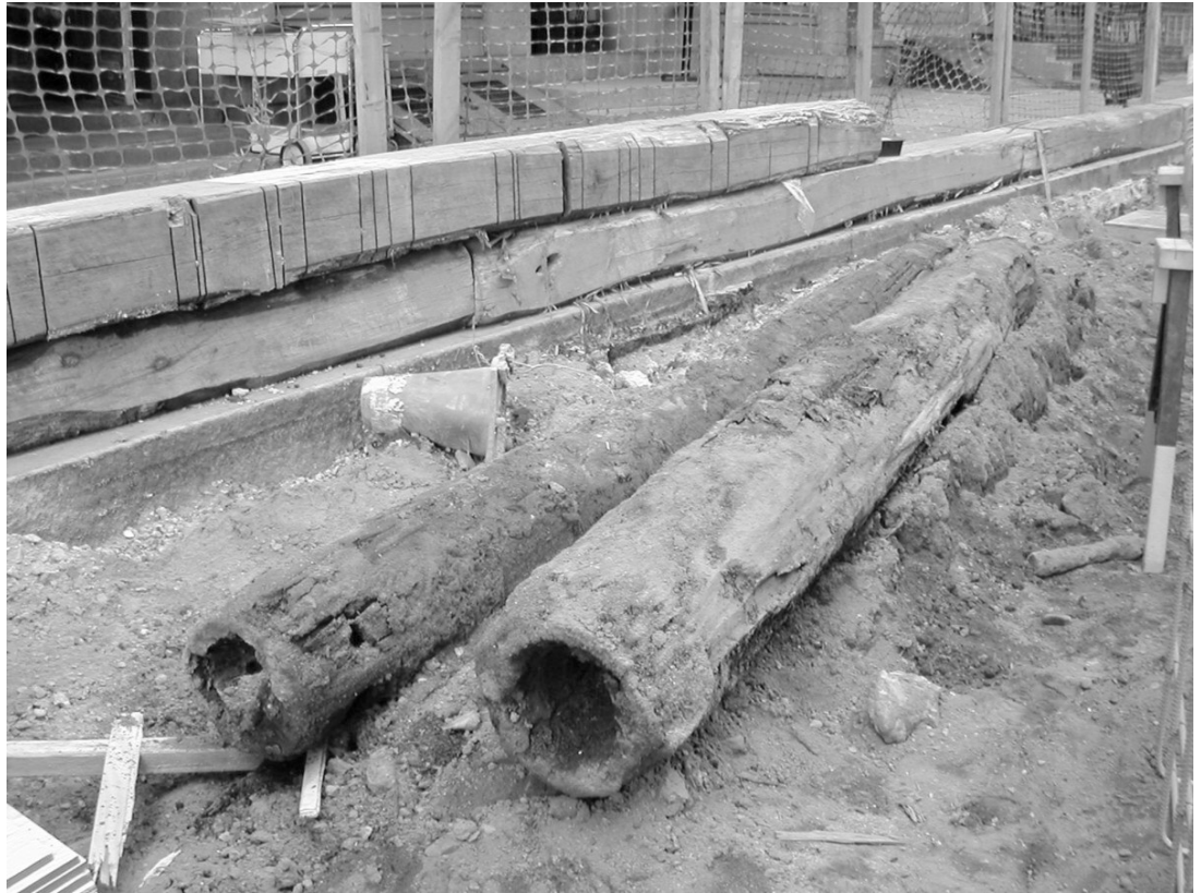
Wooden water pipes uncovered in lower Manhattan, 2004. Photo by J. Geismar, with permission.
